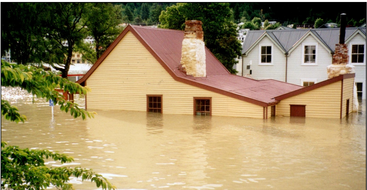
The Williams Cottage in the 1999 flood.
