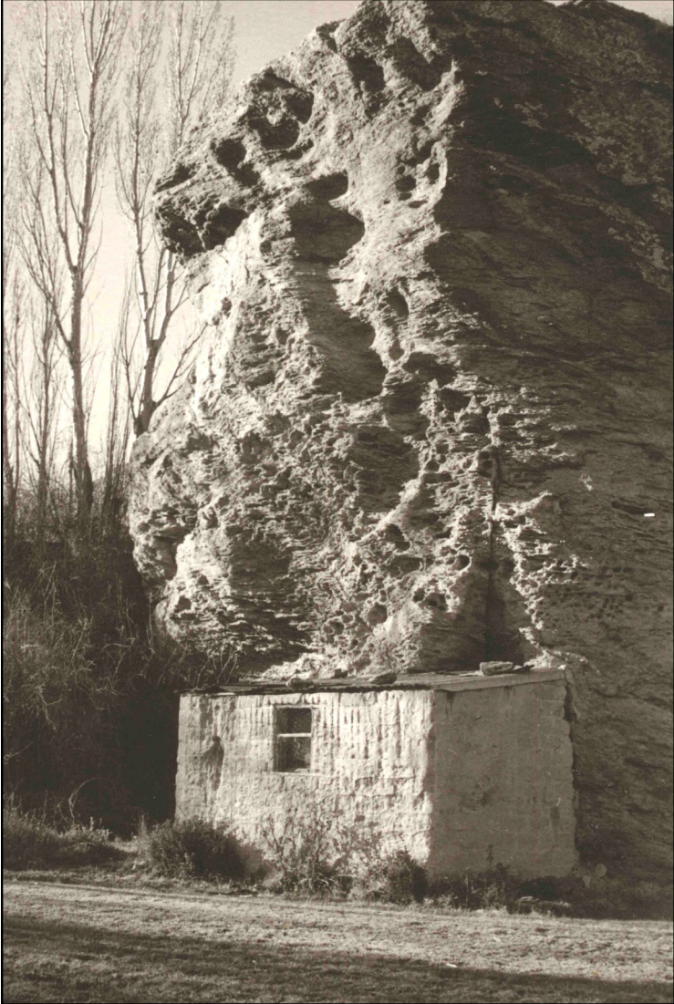
Sustainable design. Enlarged cave with wattle-and-daub extension in a sheltered location handy to transport. LDM EP0556
