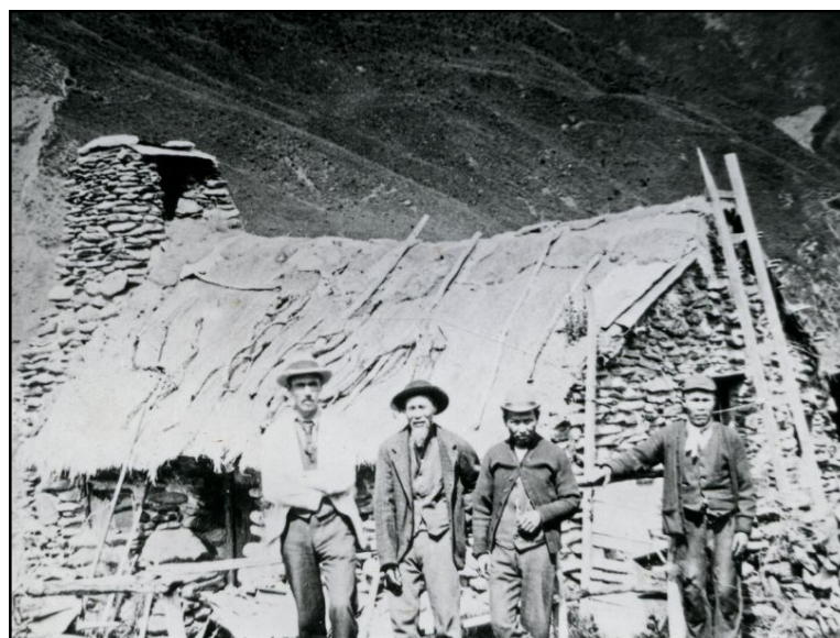
Innovative stone house with sacking roof, near Macetown. LDM EL1900
