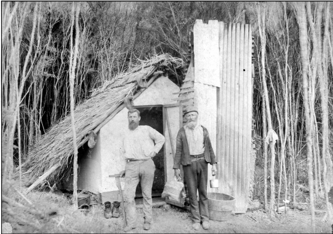
A model of mixed materials with readily-available brushwood thatch, wooden floor and chimney of imported corrugated iron, near Macetown. LDM EL4464
